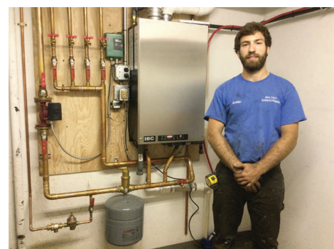
3 furnaces replacement project made possible by the Torrington Savings Bank Foundation; and the Draper Foundation and the Raymond and Gloria Oneglia Family Fund - both managed by the Northwest Connecticut Community Foundation
